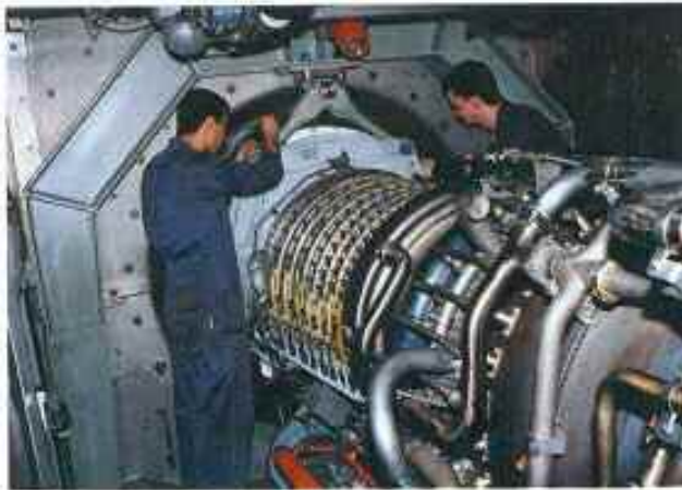
Gas turbine repairing
