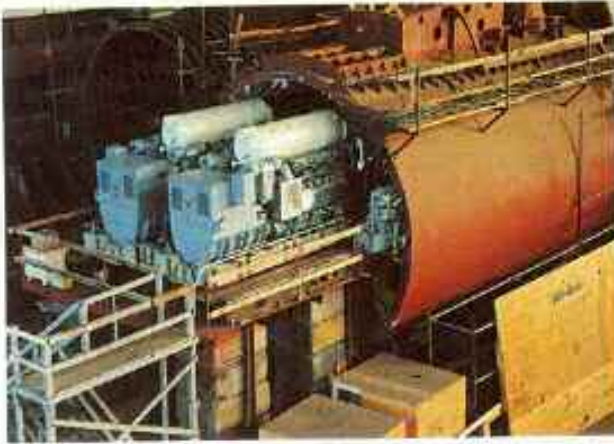
Installing the diesel generator
