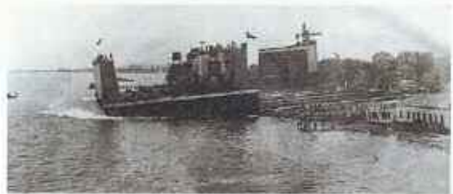
In 1926 launching of 1 st block of the floating dry-dock built for the dry-docking Ex. TCG YAVUZ
