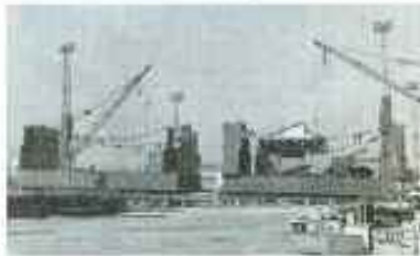
Building of dry- dock 8 in 1980
