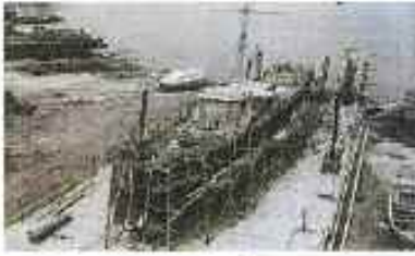
Construction of TCG KOÇHISAR in 1965
