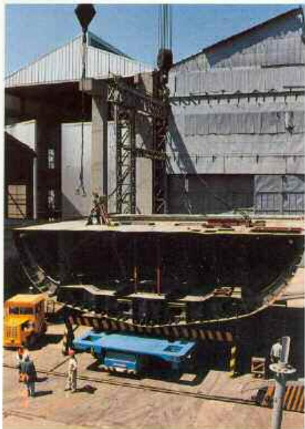
Transportation of hull module
