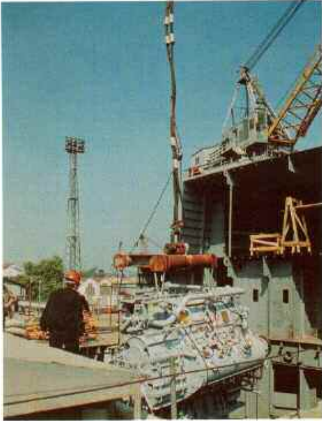
Installation of reduction gear on board.
