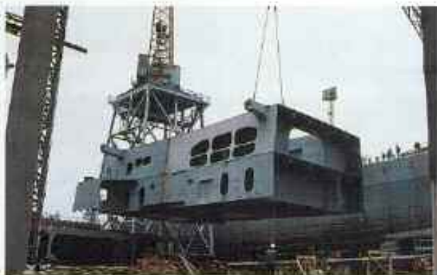
Transportation of superstructure to the slip way for mounting
