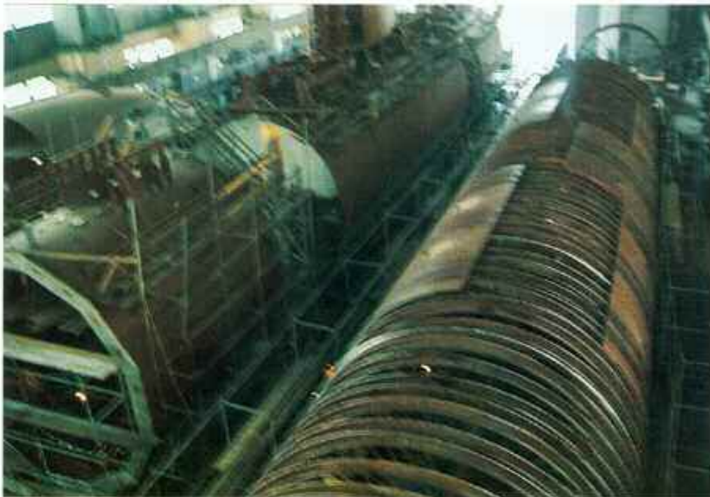
Construction of pressure hull
