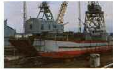
Construction of TCG Ç-150 in 1991
