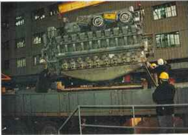
Overhauling the main propulsion of a frigate.
