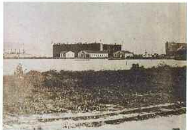
Construction of floating dry dock, 1926
