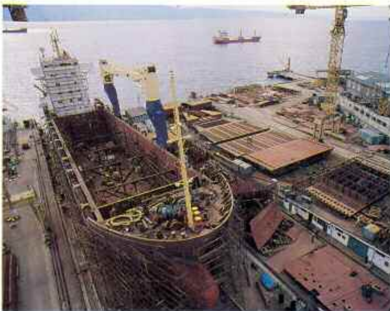
A general view over the building berths.
