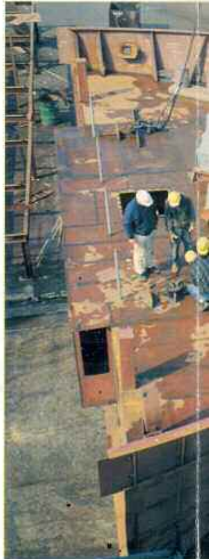
A forecabin block prior to erection.
