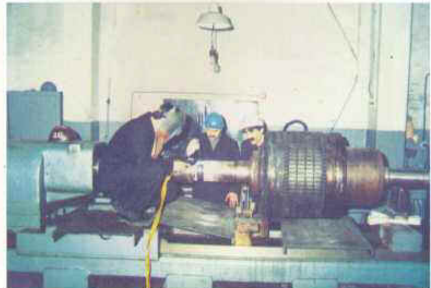
REPAIRING OF A ROTOR SHAFT
