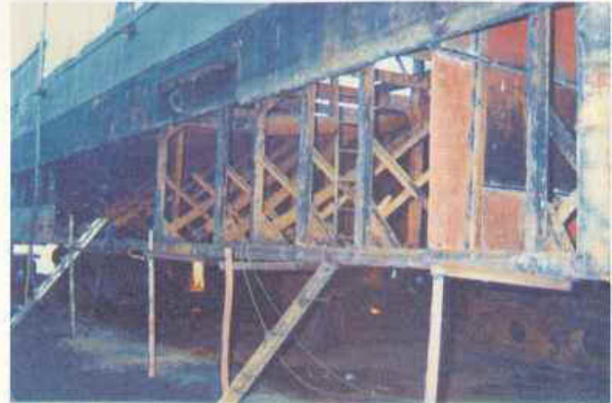
HULL REPAIR WORK ON THE FLOATING DRY DOCK
