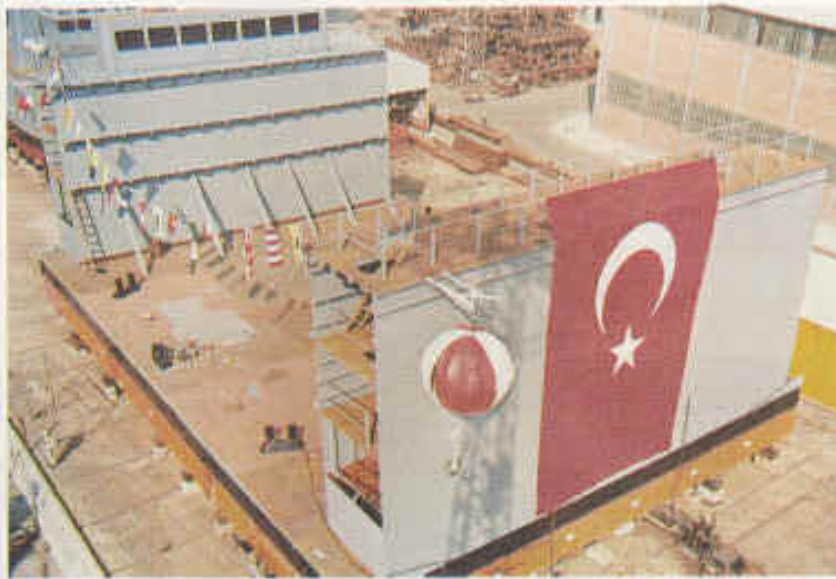
FLOATING DOCK - PONTOON BEFORE LAUNCHING
