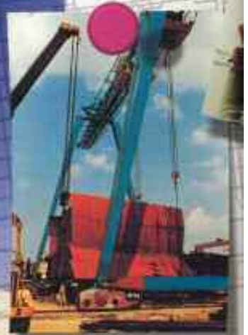
CARGO TANK NO. 7
